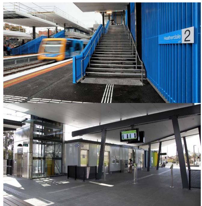
Figure 3: Railway stations built in Melbourne, Australia using prefabricated modules and other forms of off-site manufacturing (Prebuilt Pty. Ltd., 2018)
